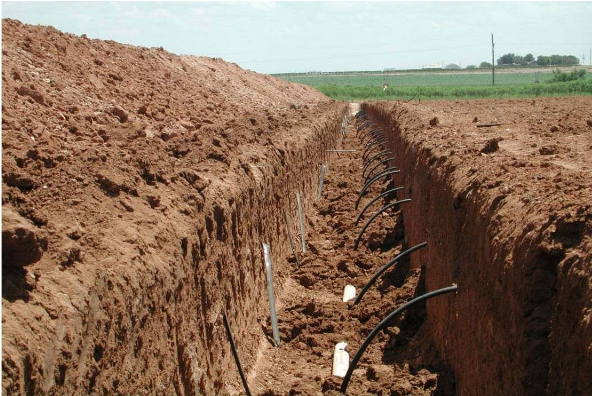
Figure 2. Drip irrigation lines recently installed in a Texas cotton field (photo courtesy of James Bordovsky, Texas A&M).
